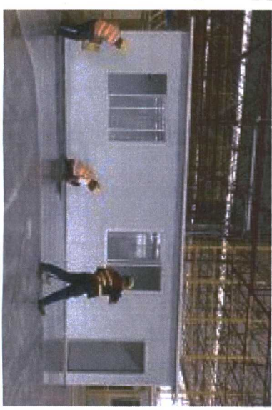
Pantiled Roof 50mm*950 Steel rock board Double sided 0.426mm Edge Colored steel bended sheet Double sided 0.426mm Window Plastic steel (1125W*1100H)
